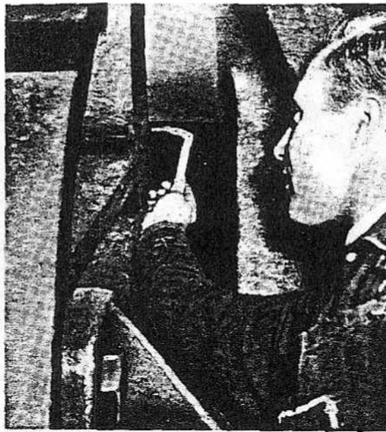
Figure 137—Testing Trunnion Clearance
